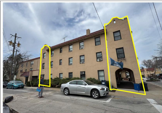
Overview of southeast façade. Concentrated concern areas are highlighted. Typically, these are below the arched caps.
